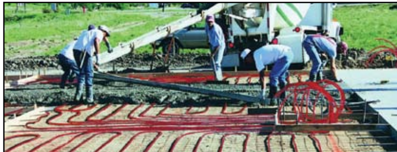
Figure 11.1 – Radiant Floor Heating Piping
